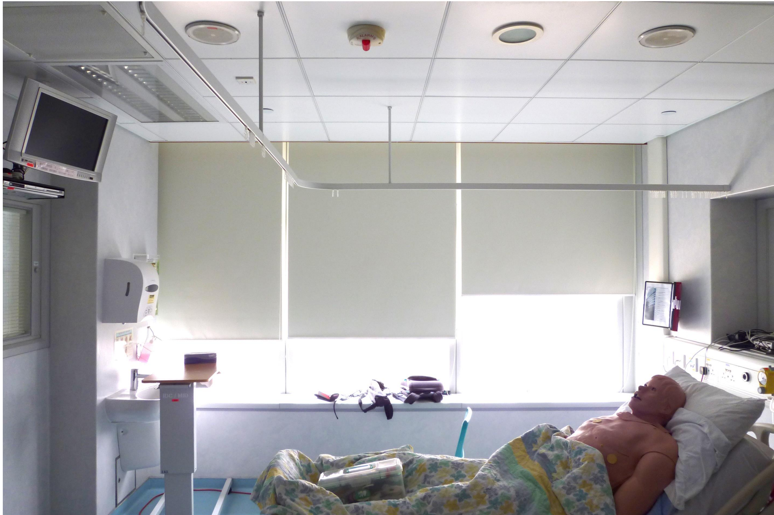
Figure: Spacious single bed patient room of isolation room A at PMH, with air supply diffusers mounted on the ceiling at the end of the patient bed and floor level exhaust underneath the head of the patient bed.
