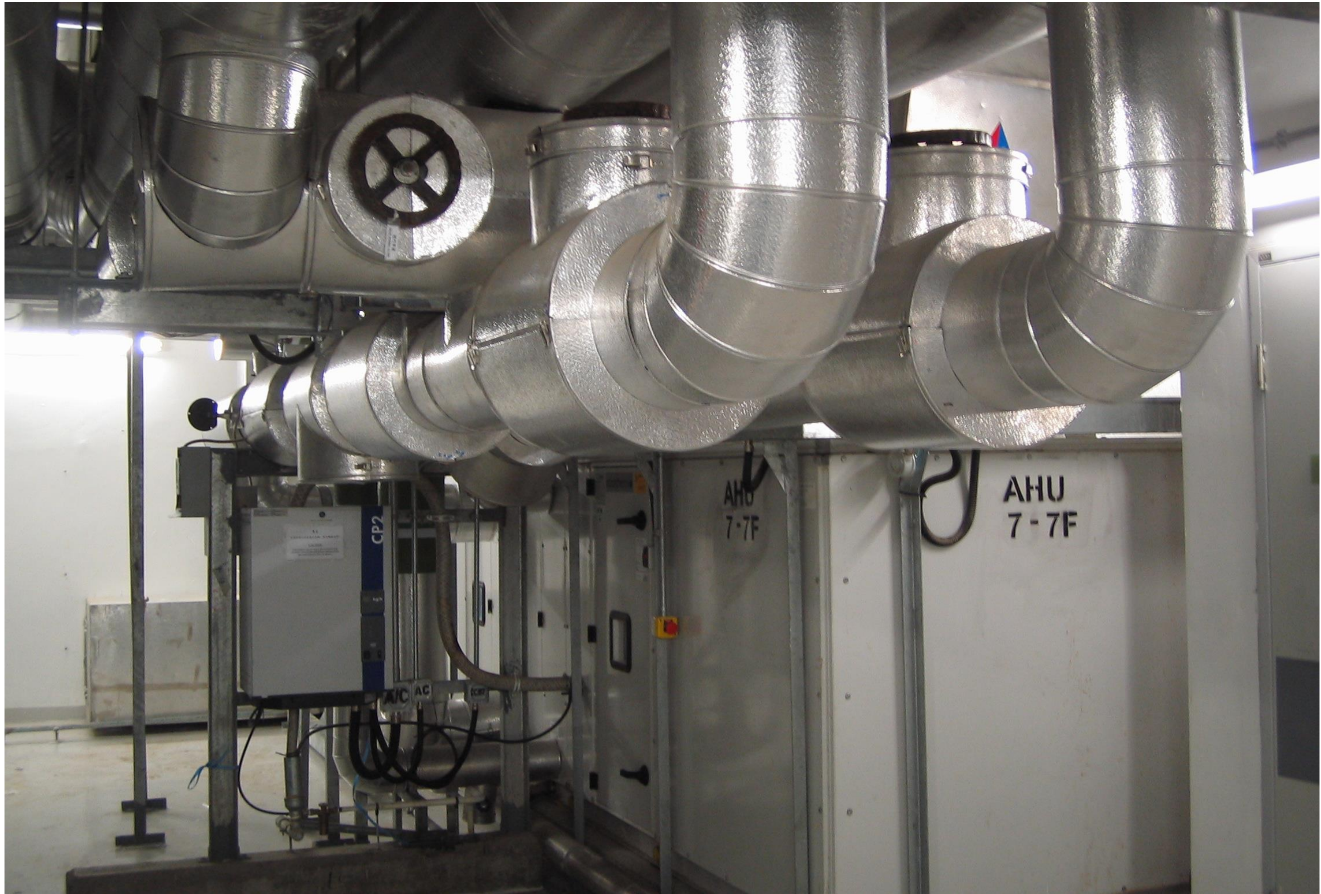
Figure: The whole 7th floor of Infectious Disease Center at PMH holds large scale mechanical Dr. Benny CHOW plants for supporting the air change and negative pressure requirements of All rooms. (ASHRAE-HKC/Med.CUHK)
