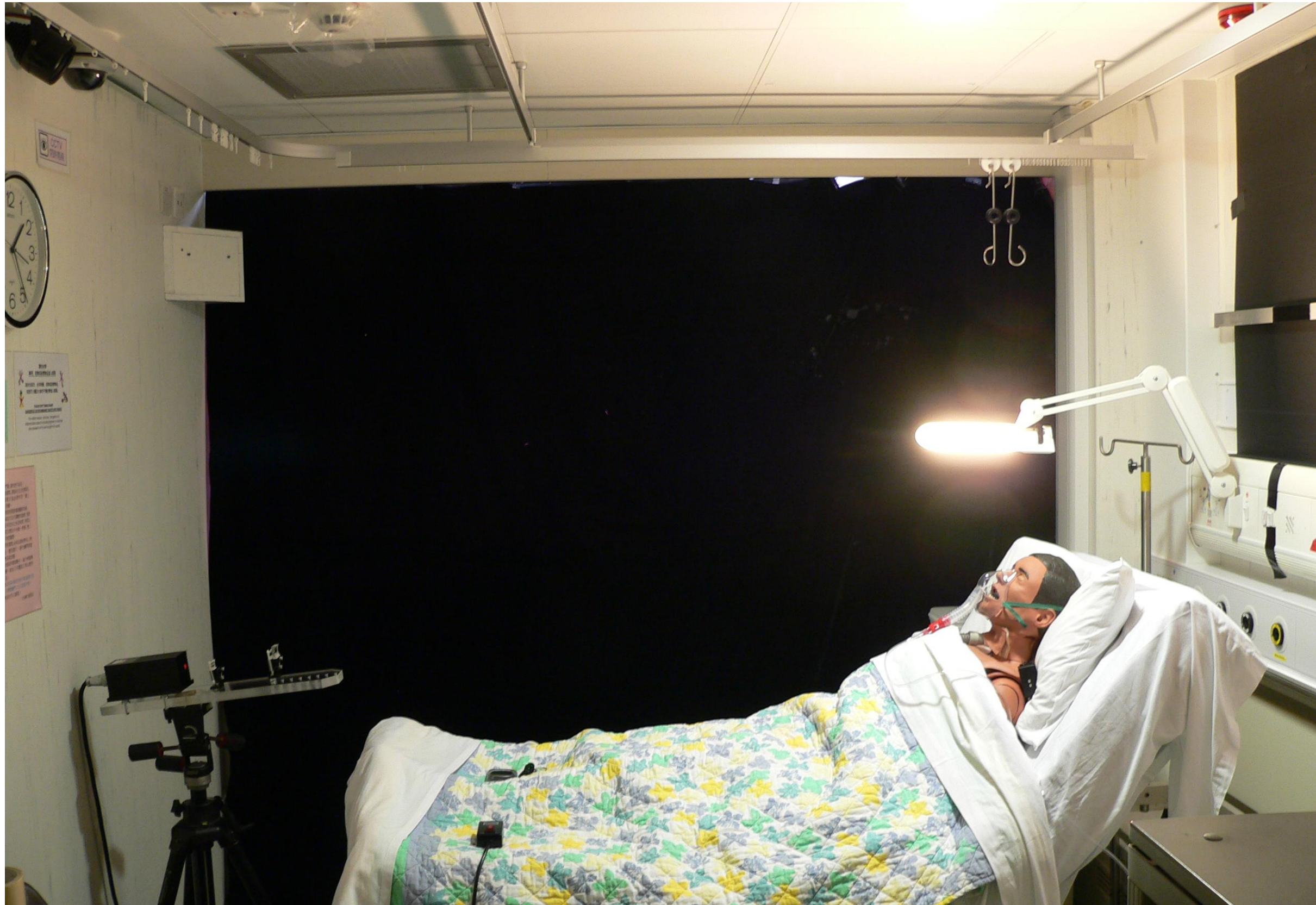
Figure: The more congested isolation room B at PWH, with air supply diffusers mounted on the ceiling at the foot of the patient bed and floor level exhausts underneath the head of the patient bed.
